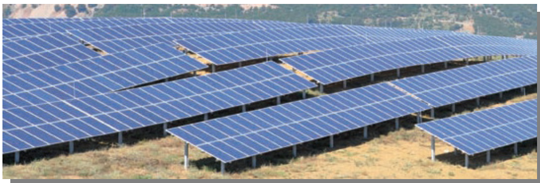
Fig. 4: Solar PV plant with crystalline Si modules and constant tilt angle
