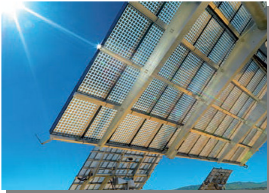
Fig. 5: Solar PV concentration technologies (CPV) – Concentrator modules with tracking systems
